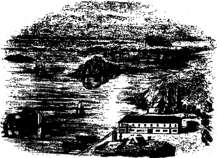
THE HARBOUR OF TRINCOMALIE FROM FORT OSTENBURG.
